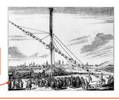
Woodcut illustration of a 46 m (150 ft) focal length Keplerian astronomical refracting telescope built by Johannes Hevelius
