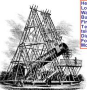
Herschel's 40 ft Telescope Location Slough, England Wavelength Optical Built 1785-9 First Light 19 February 1787 Telescope style Reflecting telescope Diameter 48 inch Focal Length 40 ft Mounting Alt-azimuth.
